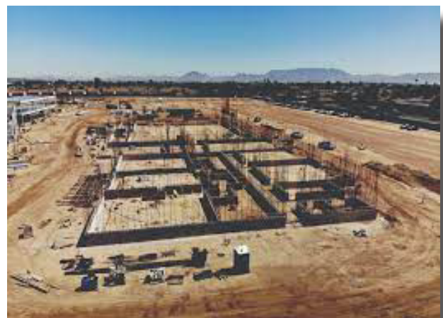
Camino Del Sol High School construction work
